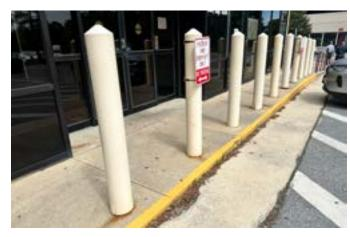
Figure 58 - Damaged Bollard Covers
