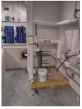
The boiler (left) and domestic water heat exchanger (right) remain condition. However, HVAC equipment exceeding 20 years of age is nearing the end of its useful life, despite regular maintenance,
