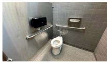
Figure 79 - Missing Vertical Grab Bars
