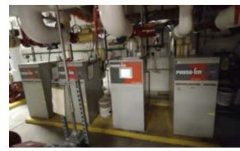
Figure 20 - Lochinvar Gas Fired Boilers
