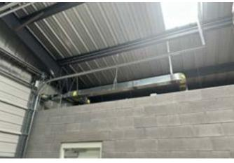
Figure 106 - Ventilation Ductwork
