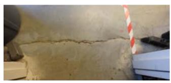
Figure 143 - Example of Floor Crack
