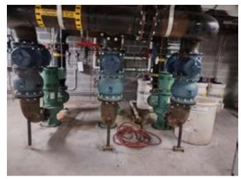
Figure 48 - Condenser Water Pumps
