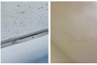
Figure 40 - Cracking Sealant Figure 41 - Water Damaged Ceiling
