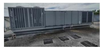
Figure 63 - Packaged RTU
