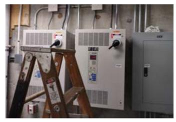
Figure 96 - Variable Frequency Drives
