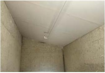
Figure 84 - Absence of Fire Stopping in Stairwell
