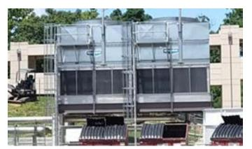
Figure 23 - Cooling Towers
