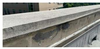
Figure 121 - Chipped CMU Barrier Sealant
