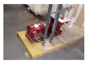
Figure 95 - Circulating Pump
