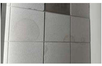
Figure 73 - Ceiling Tile Water Spots
