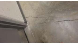
Figure 43 - Cracked Concrete
