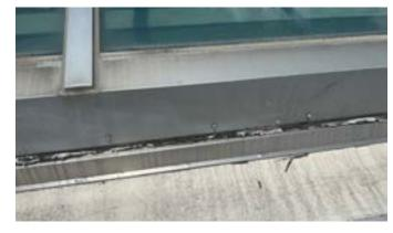
Figure 32 - Cracking Sealant at Skylight
