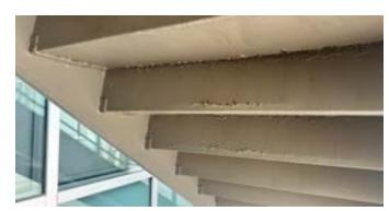
Figure 6 - Corrosion and Peeling Paint
