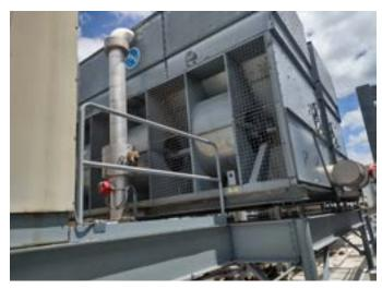
Figure 35 - Cooling Tower
