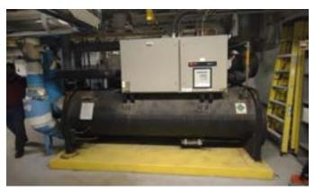
Figure 21 - Water Cooled Chiller
