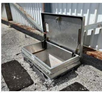
Figure 66 - Roof Access Hatch Without Safety Railings
